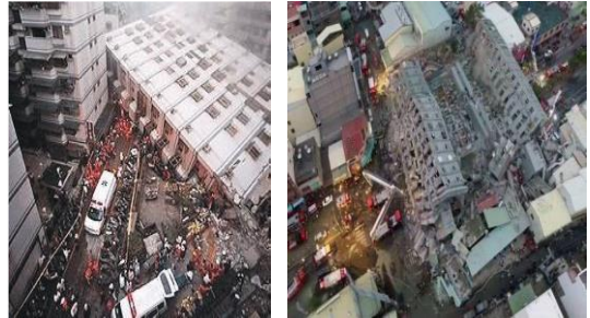
Figure 9: Full blockage by RCC buildings
