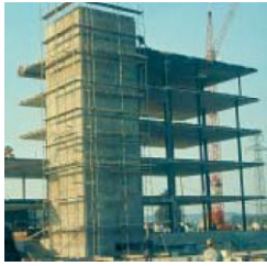
1. Torsional Irregularity
