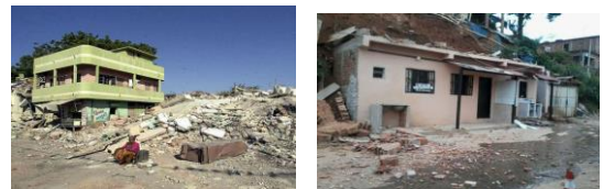
Figure 4: Collapsed RCC buildings
