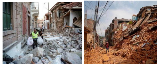
Figure 8: Full blockage by URM buildings
