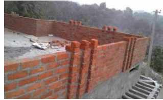
Unsupported Parapet
