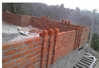
Figure 13: Unsupported Parapet
