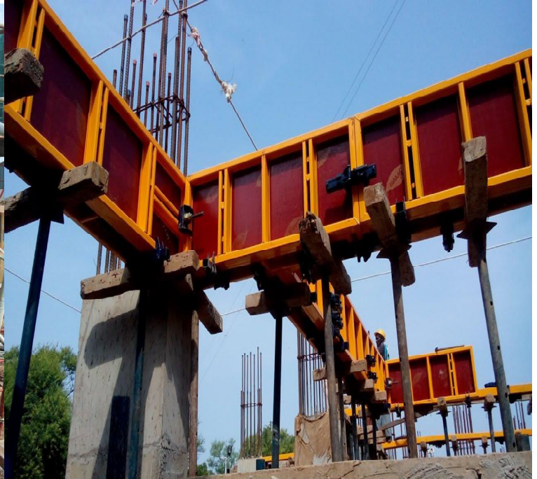
Steel formwork with horizontal supports of a beam to ensure safety
