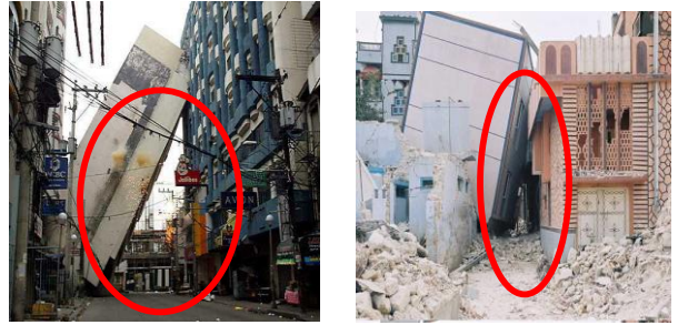
Figure 7: Partial blockage by RCC buildings according to second condition
