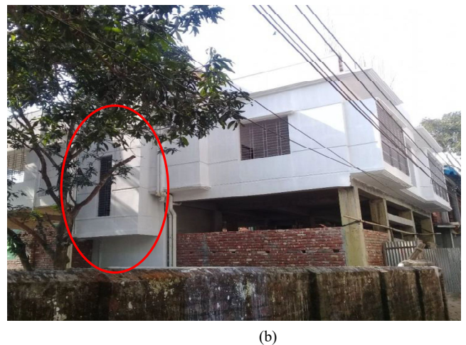
Figure 3: Short column due to a) reduced height, b) partially infill walls
