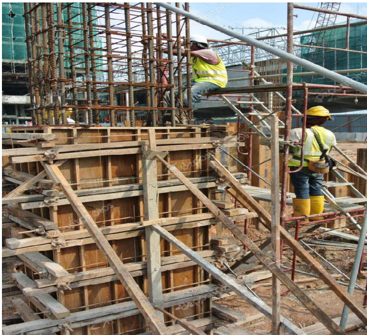
Timber formwork with vertical supports of a column to ensure safety
