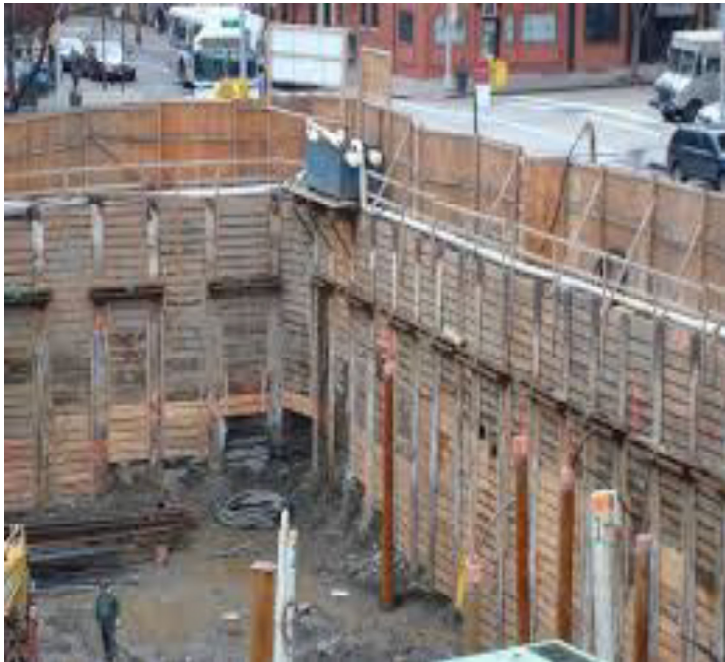
Protection of adjoining building
