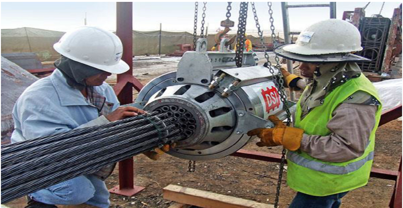
Tensioning operation is being conducted using protection
