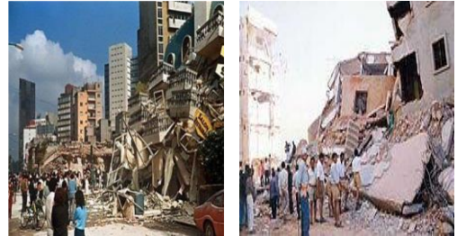
Figure 5: Partial blockage by URM buildings
