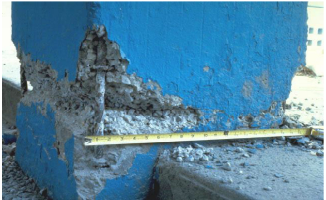
Figure 11: Poor concrete quality
