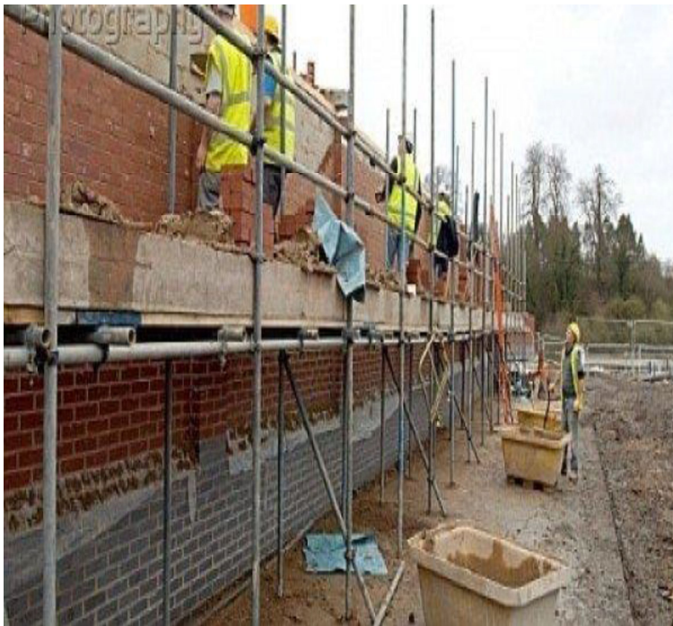
Scaffold during construction of walls to ensure safety of workers
