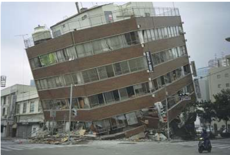
Photo 3.1: Tilting of expressway and buildings during Kobe earthquake in 1995
