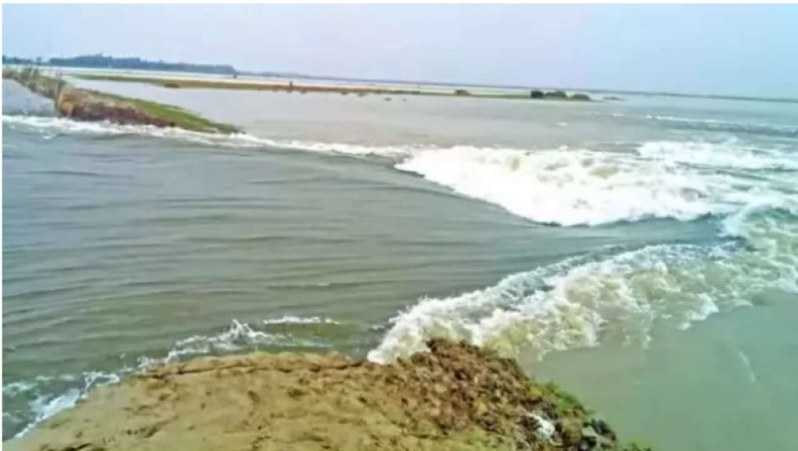
Photo 5.1: Polder breached at Koyra, Khulna during Cyclone Amphan
