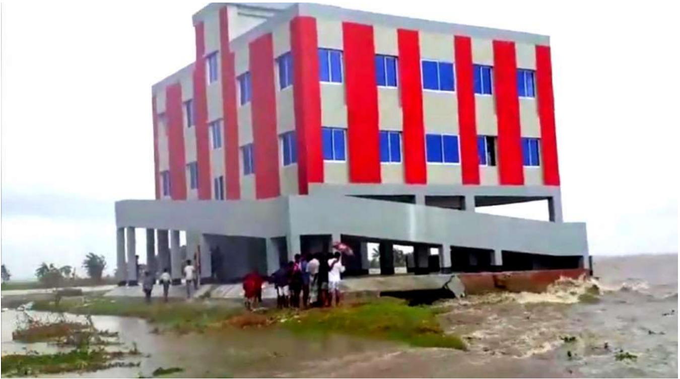
Photo 5.2: A newly constructed school building being washed away by flood and erosion of Padma River in July, 2020
