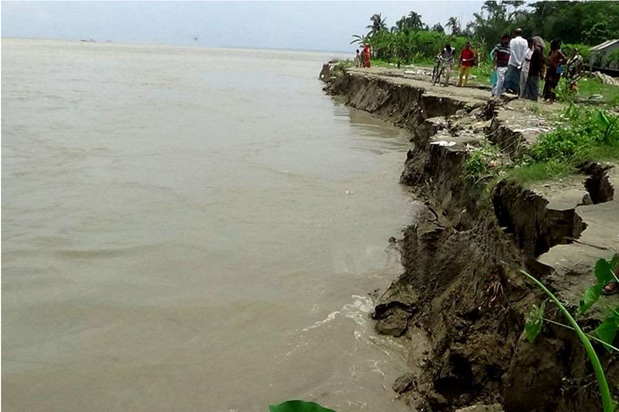
Photo 3.3: Typical scene of bank erosion of Padma river
