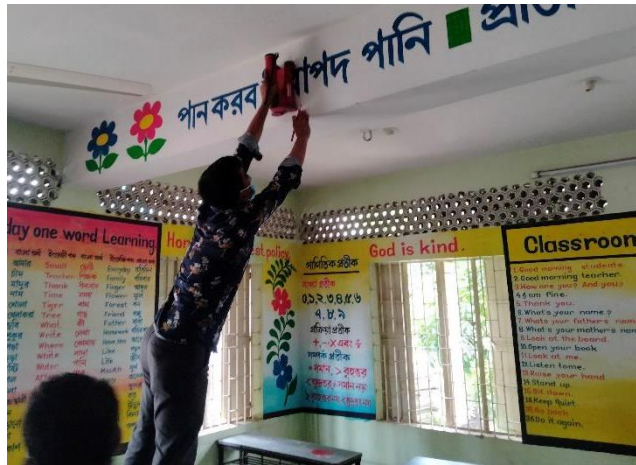
Figure 5.1: Ferro-scanning of a beam
