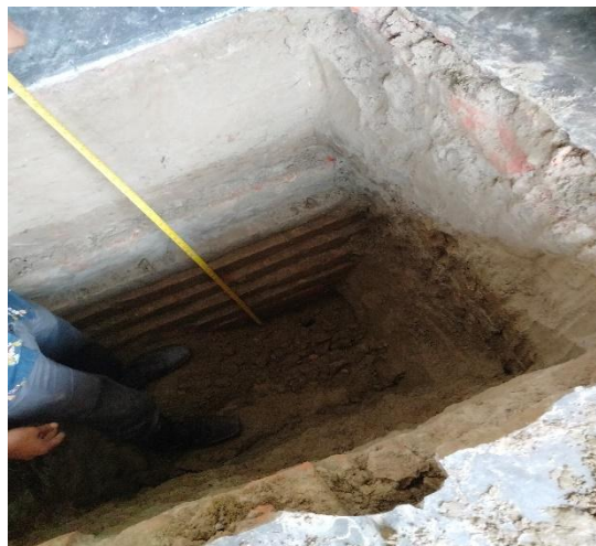
Figure 5.1: Footing Excavation
