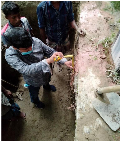
Figure 5.2: Footing excavation
