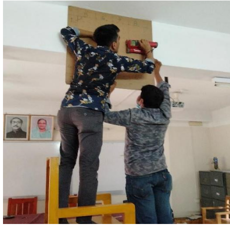
Figure 5.1: Ferro-scanning of a beam
