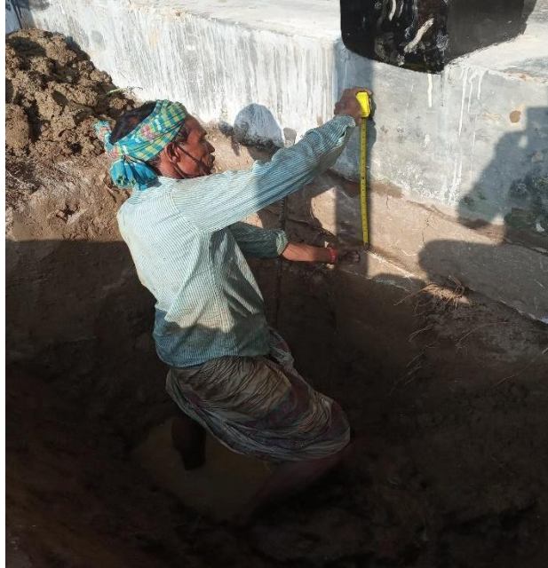
Figure 5.1: Footing excavation
