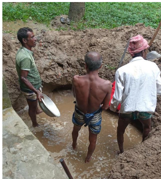
Figure 5.2: Footing excavation
