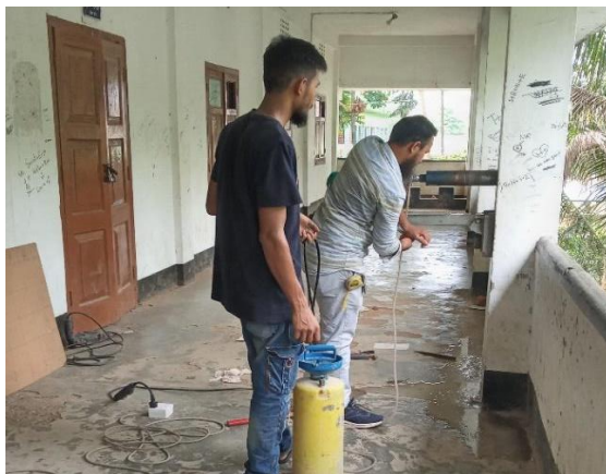
Figure 5.1: Core extraction from a column
