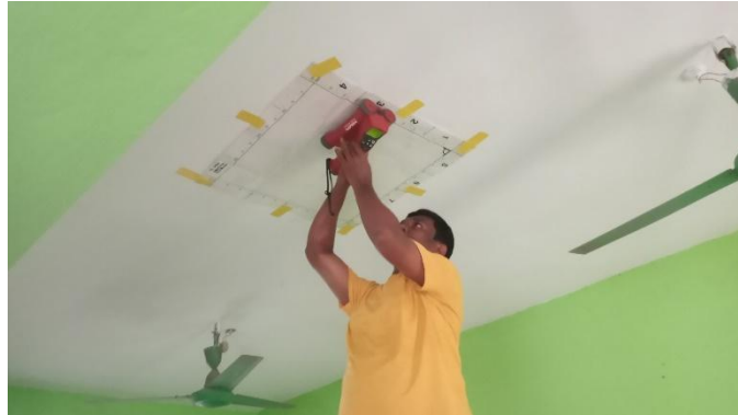
Figure 5.1: Ferro-scanning of slab
