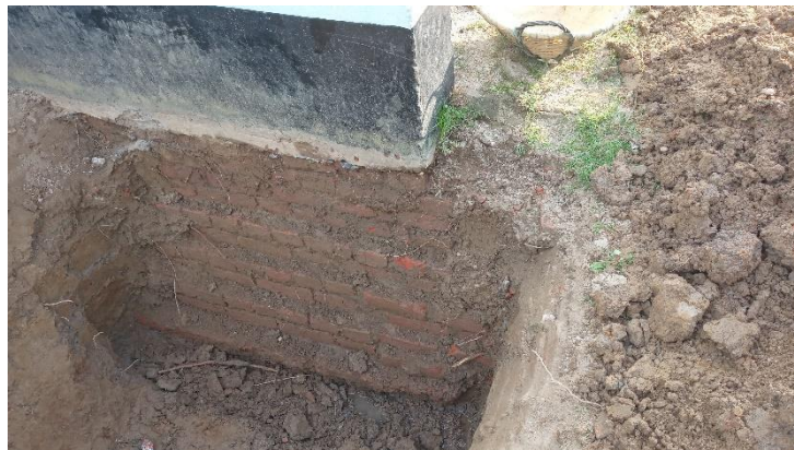
Figure 5.2: Footing excavation
