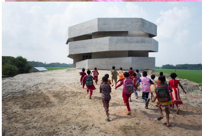
Picture 6: Multi-purpose cyclone shelter built by NGO
