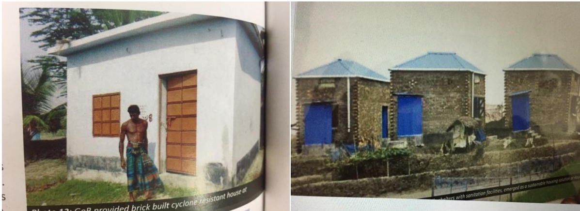
GoB Brick-built cyclone resistant house
