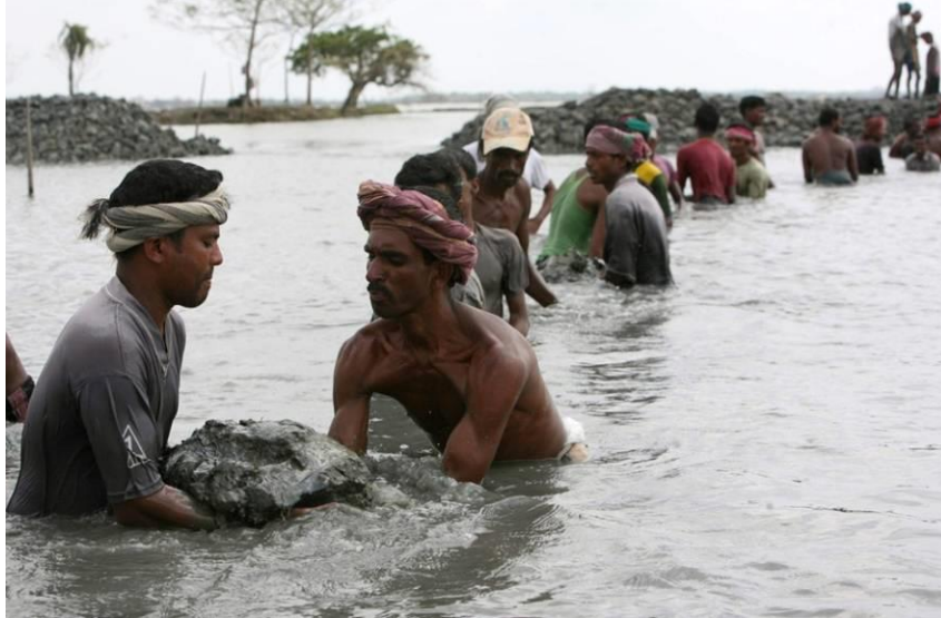
Picture 3: During post-Aila the villagers started rebuilding the breaches with their own hand
