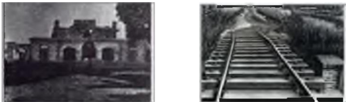
Figure 1.4: Damage of building in 1897 earthquake and damage of rail track in 1997 earthquake
