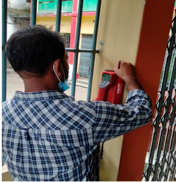
Figure 5.1: Ferro-scanning of a column
