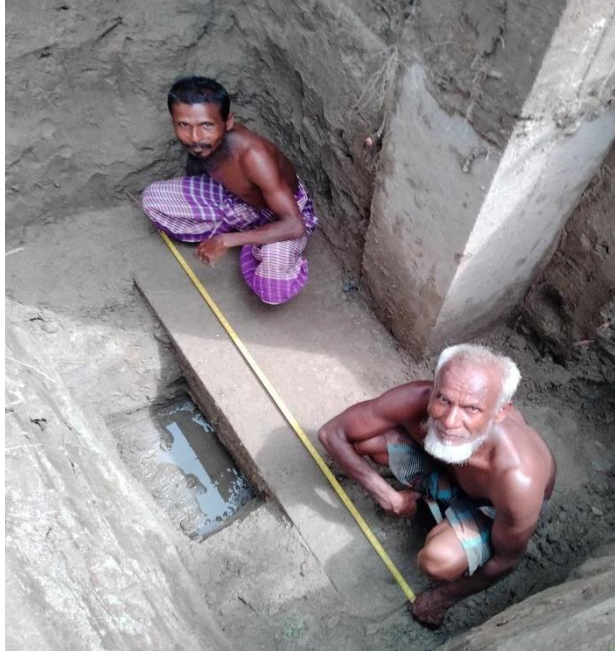
Figure 5.1: Excavation of footing
