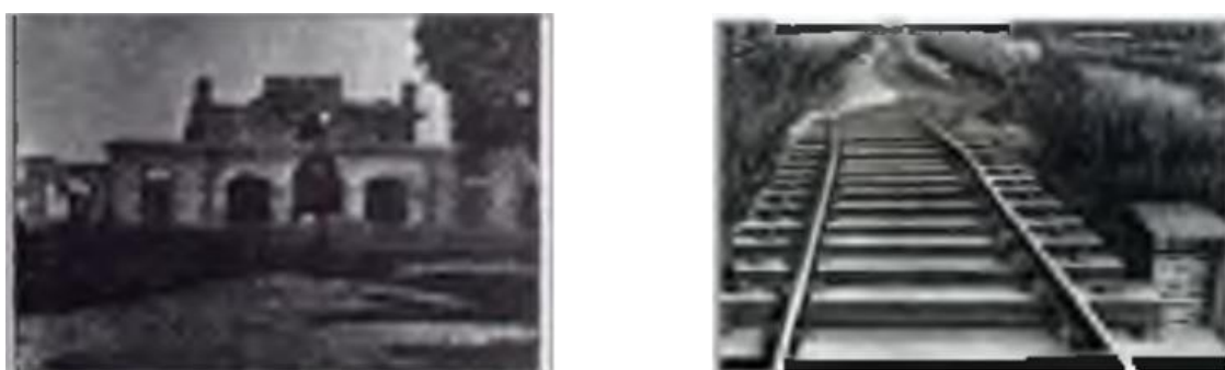
Figure 1.4: Damage of building in 1897 earthquake and damage of rail track in 1997 earthquake
