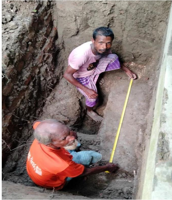
Figure 5.1: Footing excavation
