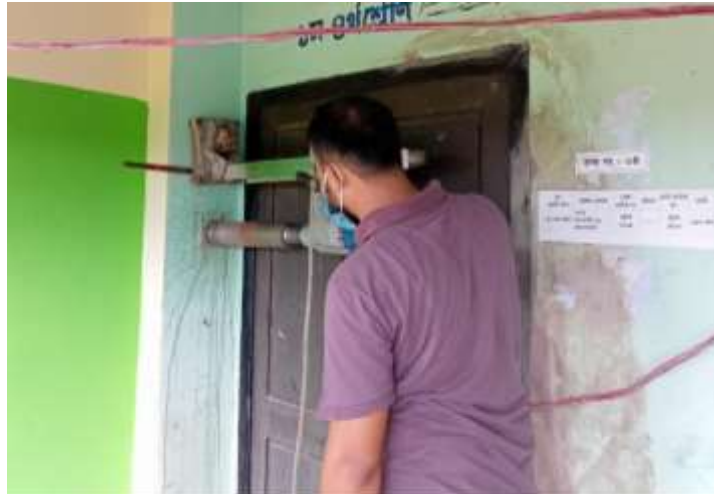
Figure 5.1: Core extraction from a column
