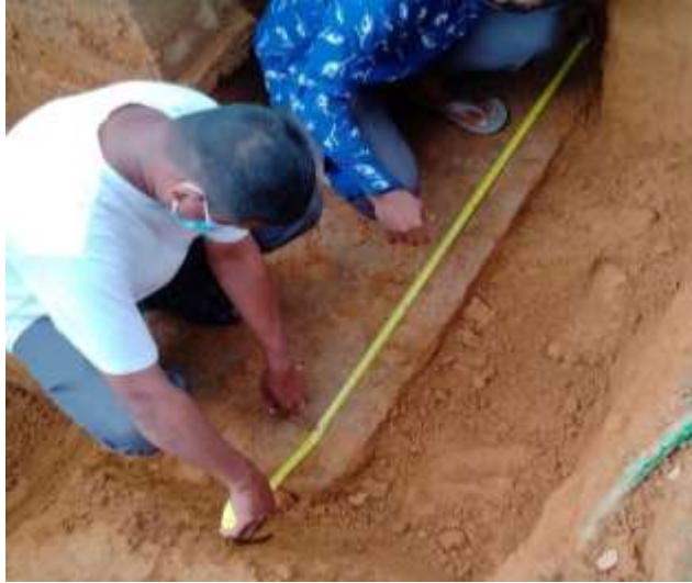
Figure 5.3: Footing excavation
