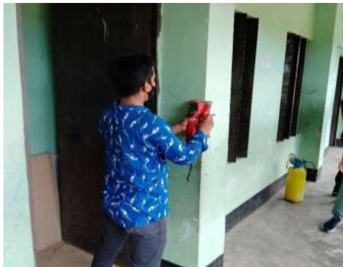
Figure 5.2: Ferro-scanning of a column
