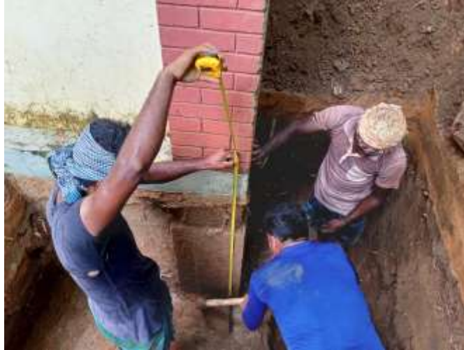
Figure 5.3: Footing excavation
