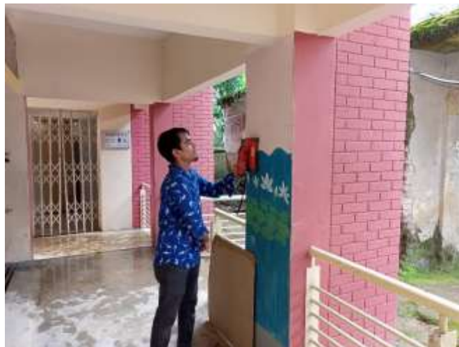
Figure 5.2: Ferro-scanning of a column
