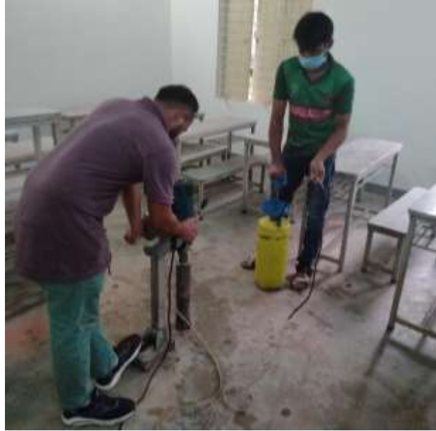
Figure 5.1: Core extraction from slab
