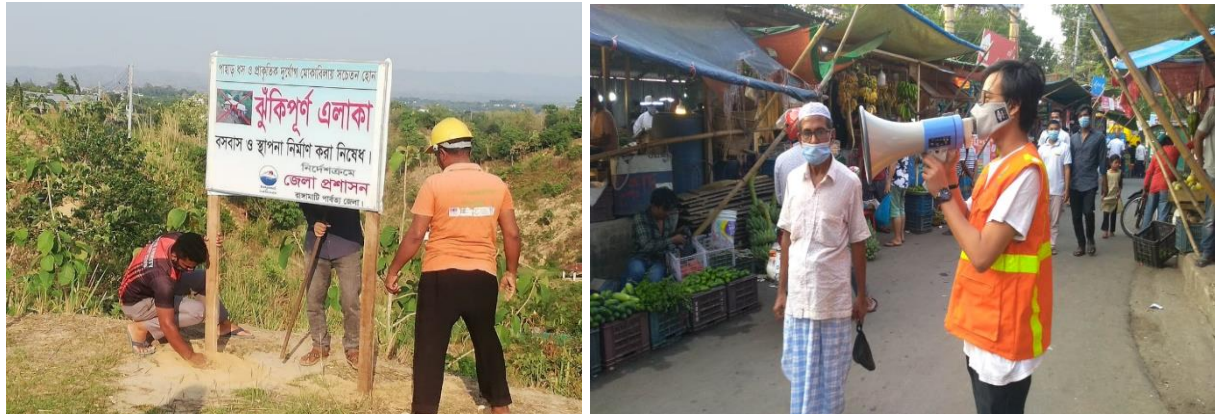
Figure 6: Volunteers are in action: Installation of Billboards at landslide hotspots in Rangamati (L), dissemination of Covid-19 awareness message in Tangail (R)
