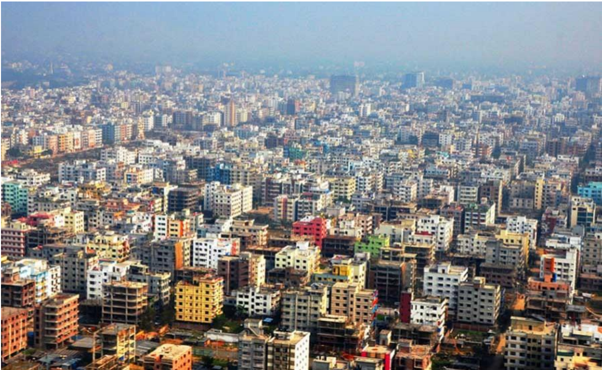
Figure 1: Mushrooming growth making city vulnerable to earthquake (file photo)
