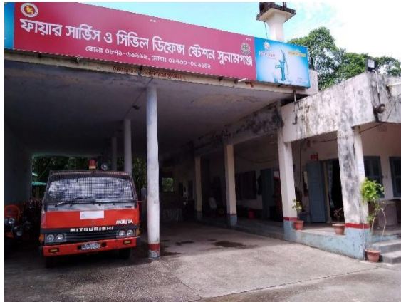
Fire Service & Civil Defense Station
