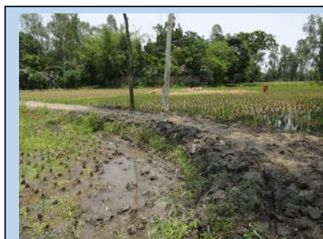
EGPP Supported Earthen Rural Road at Islampur, Jamalpur
